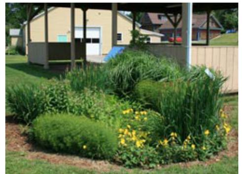
The rain garden above, shown at installation (L) and a few years later (R) captures roof and yard run-off. By slowing water down, it provides stormwater flood control and filters out pollutants. Photos: Connecticut Sea Grant
