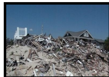
Destruction from Sandy in Mantoloking, NJ. Image: New Jersey Sea Grant
