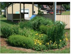
The rain garden above, shown at installation (L) and a few years later (R) captures roof and yard run-off. By slowing water down, it provides stormwater flood control and filters out pollutants. Photos: Connecticut Sea Grant
